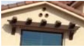
Wood and rafters
