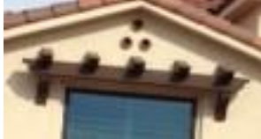
Wood and rafters
