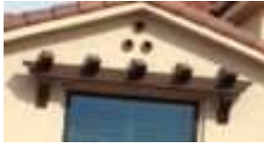
Wood and rafters
